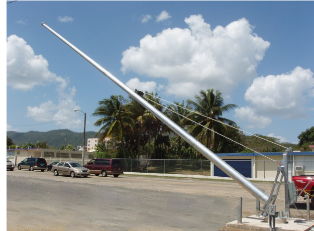
ARE's Vertical Gin Pole supports turbines up to a 50' pole height
